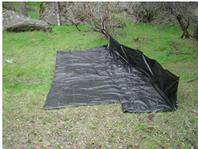
Figure 4.1. Installation of geotextile sediment trap and apron.
